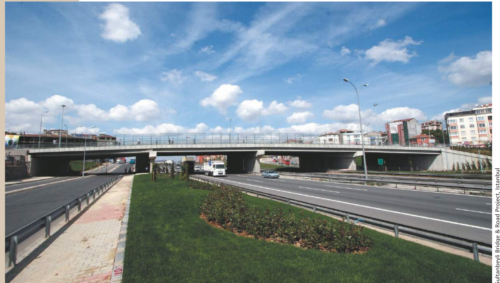
Sultanbeyli Bridge & Road Project, Istanbul
