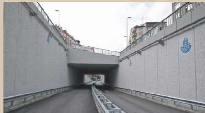
Kağıthane Inferior Passage, Road & Infrastructure Project, Istanbul
