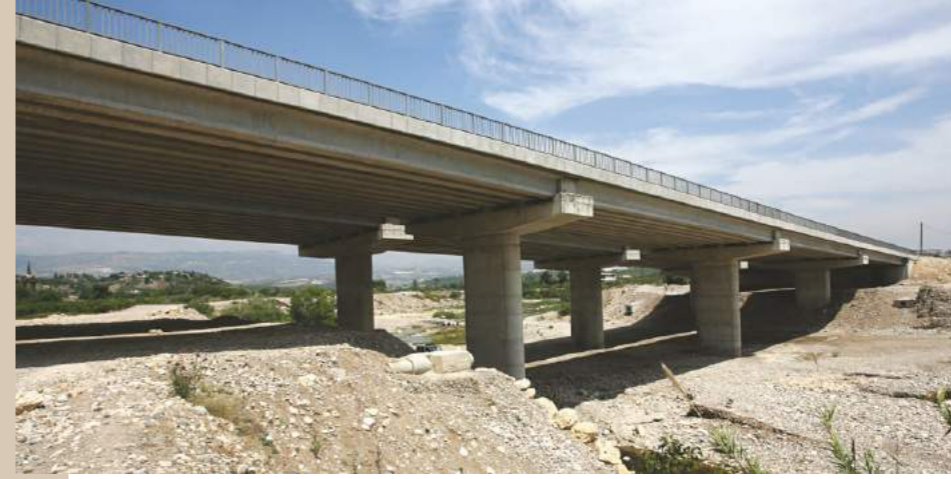
13 th st.'s Bridge Construction, Mersin
