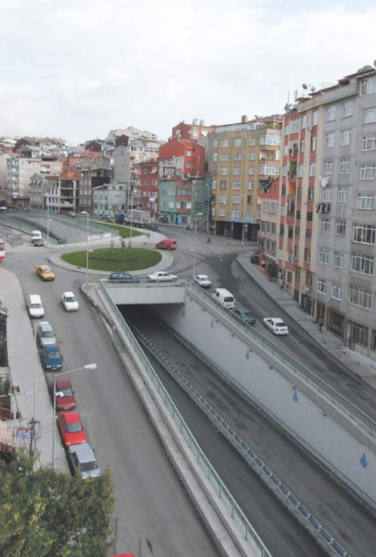
Kağıthane Inferior Passage, Road & Infrastructure Project, Istanbul
