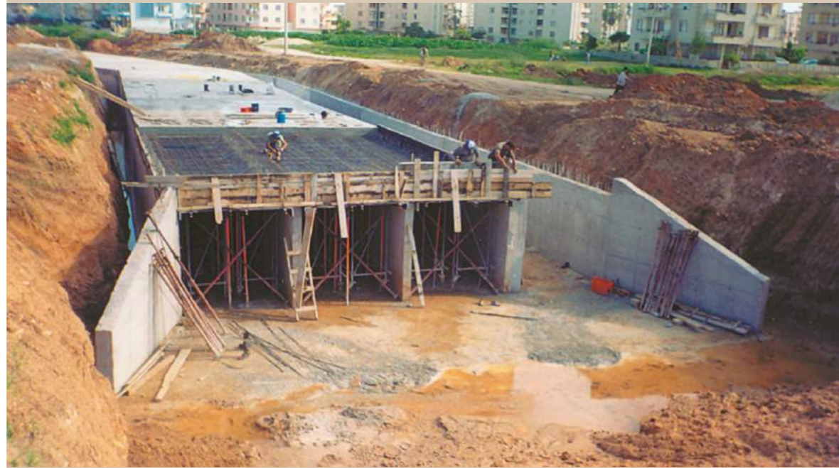
Storm water line, Mersin
