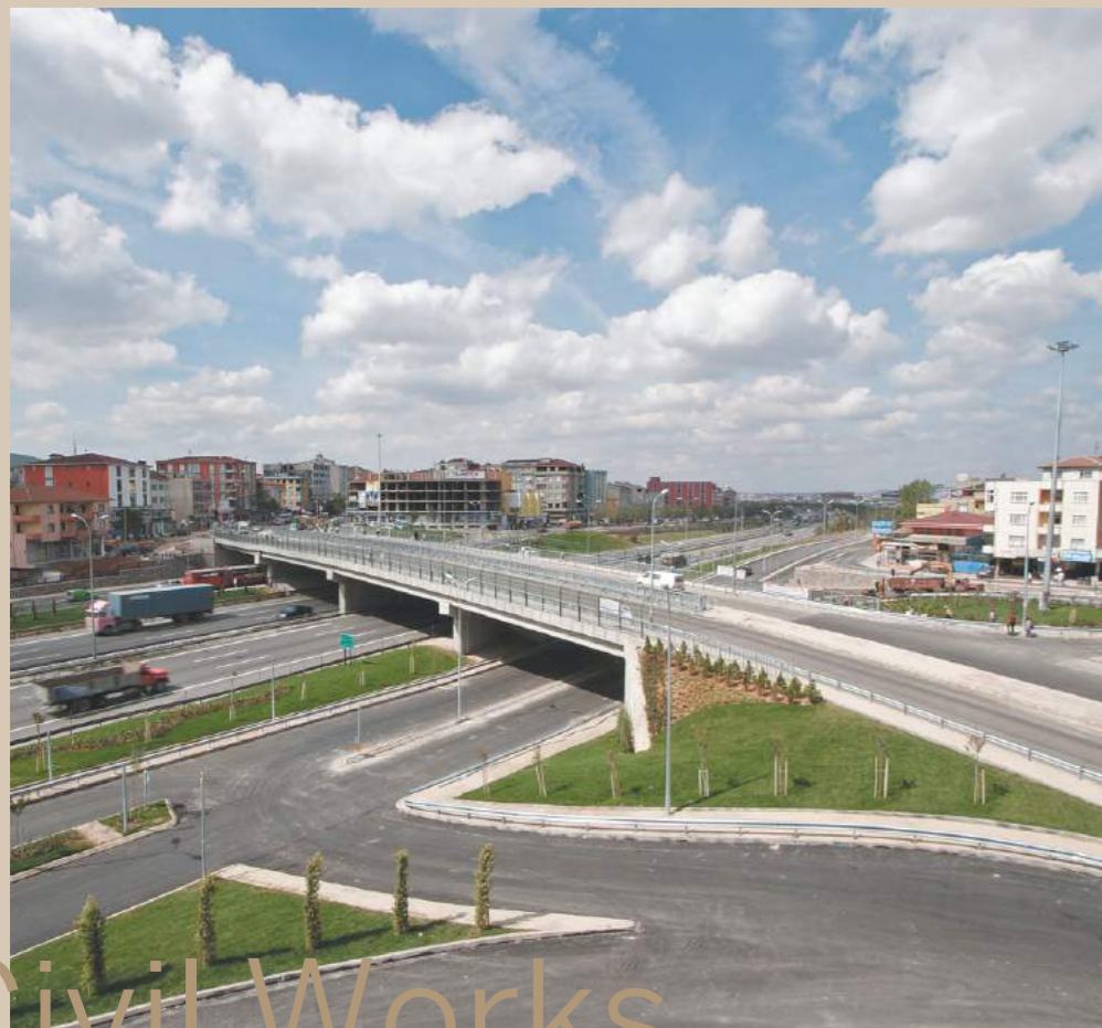
Sultanbeyli Bridge & Road Project, Istanbul
