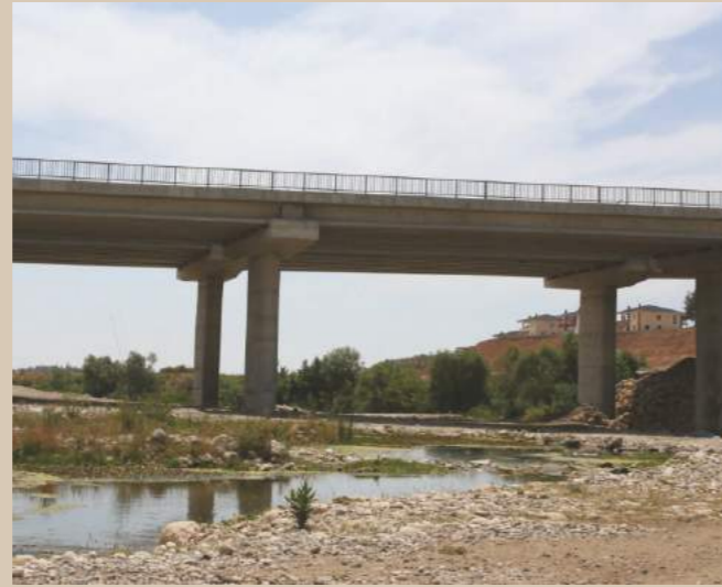
13 th st.'s Bridge Construction, Mersin
